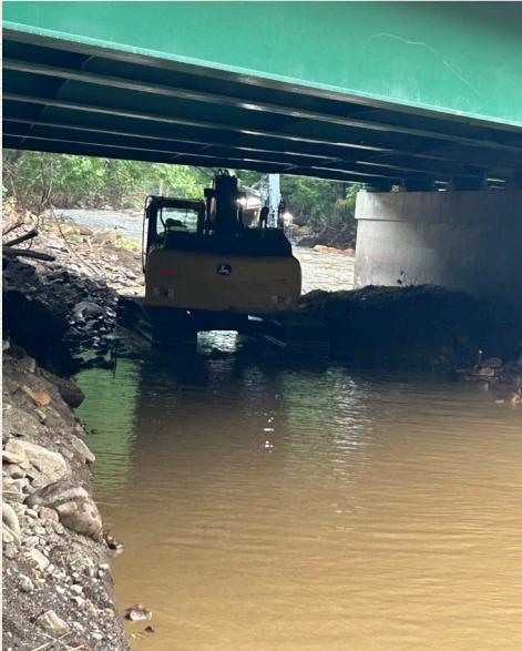
Woody debris upstream of bridge and lodged under bridge significantly diminished flow capacity, could cause bridge to overtop. SHA is repairing south abutment of bridge and scour area. USGS will place new Georges Creek stream gage on bridge span now that area has been cleared of debris.
